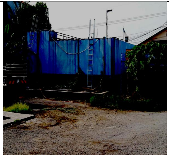
Waste Treatment Plant
