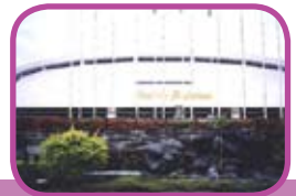
Sarawak Outdoor Stadium
